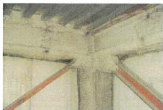
吹付け材の例(梁・柱)
